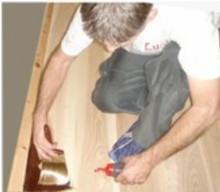
Use a 175 rpm buffer with a **red pad**. Initially, squeeze sufficient oil on the pad to get an easy start. Then spread the oil parallel with the planks using a minimum amount of oil. Buff the floor once more without adding any oil in order to even out the application.
