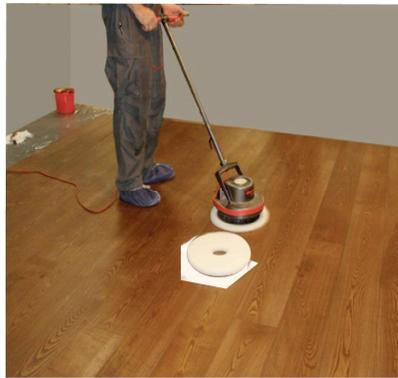
**There is no need to apply a second layer on top of the Monocoat Oil because this extra layer will not bond with the primarily bonded Monocoat layer.**
